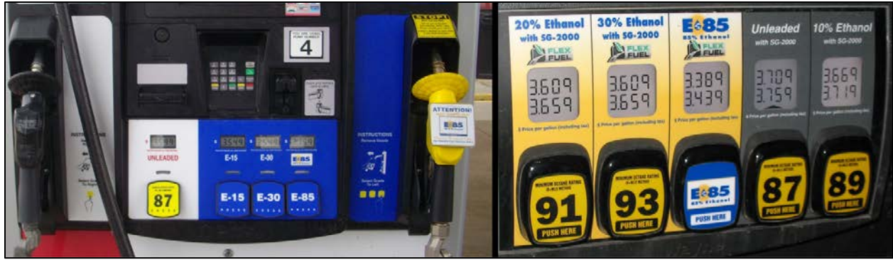
Figure 11. Two fuel configurations at ethanol blender pumps
