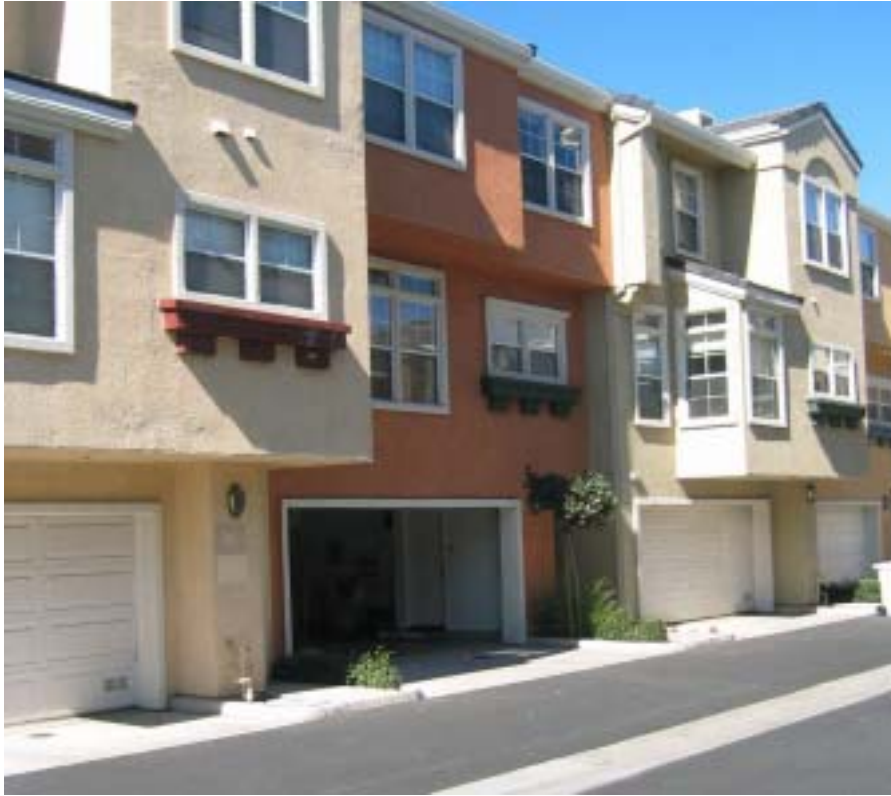
Figure 5-8. The ACH of this condominium garage in Fremont, California, was measured
