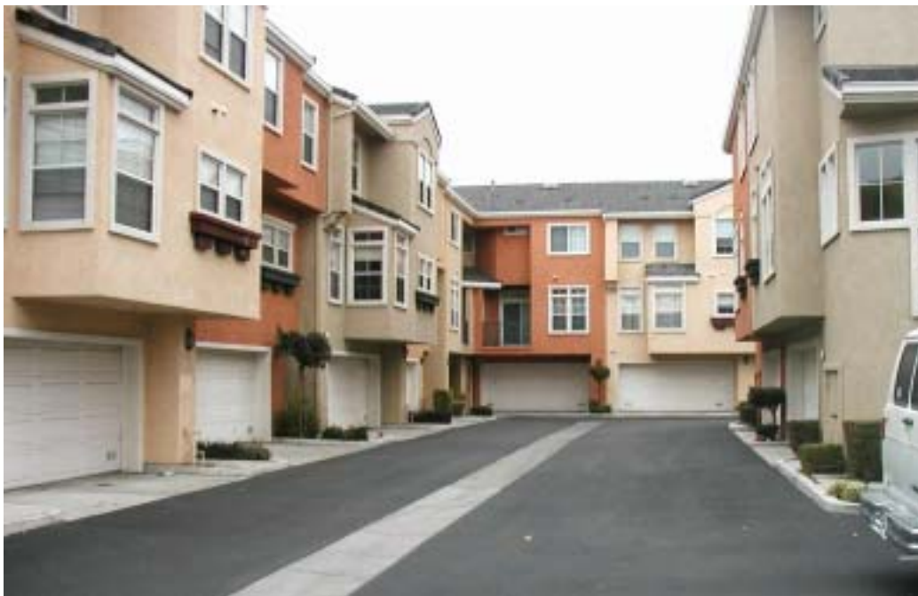
Figure 5-9. The Fremont, California, garage had substantial wind-shielding due to the “canyon-like” configuration of the condominium complex
