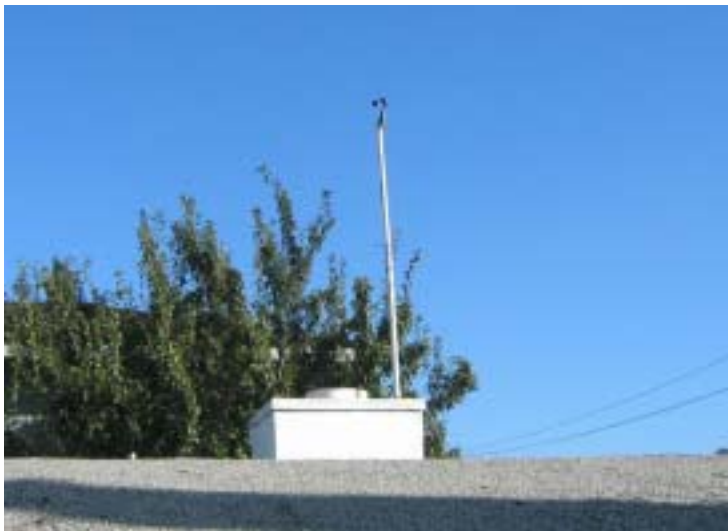
Figure 5-4. An anemometer is usually installed high on the building roof to measure wind speed
