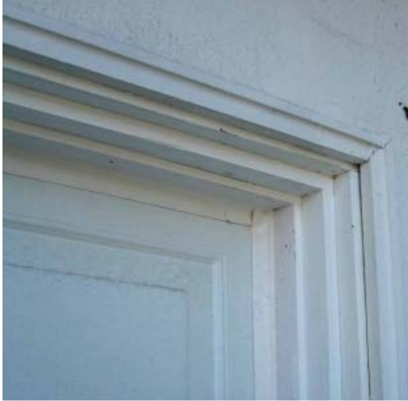
Figure 5-12. The San Jose garage was selected because the door was sealed by vinyl flaps, which were anticipated to provide a low ACH
