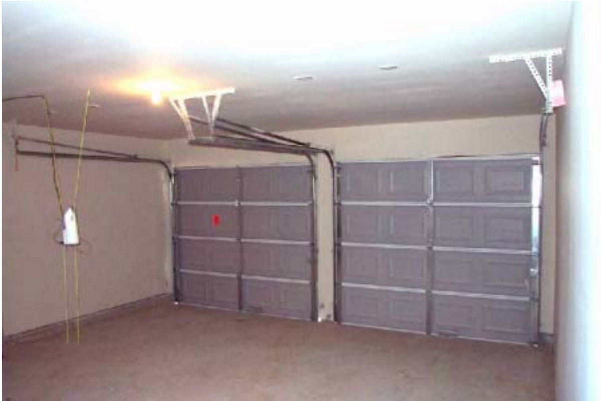
Figure 5-6. The Spring, Texas, house is a new home with an attached two-car garage
