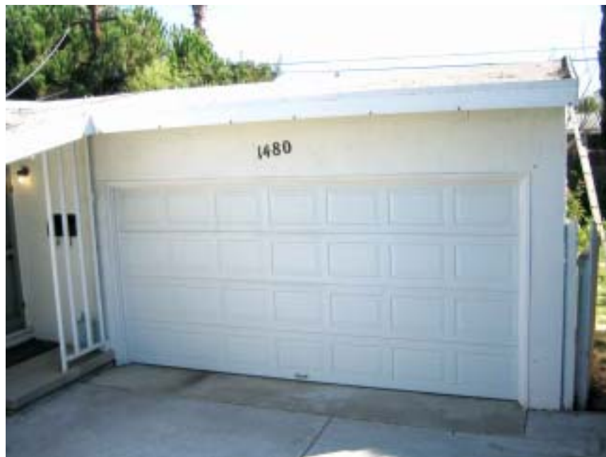
Figure 5-11. The ACH of this attached two-car garage in San Jose, California, was measured
