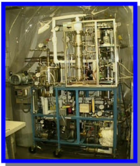
Figure 7. Epyx fuel processor and LANL PROX.
