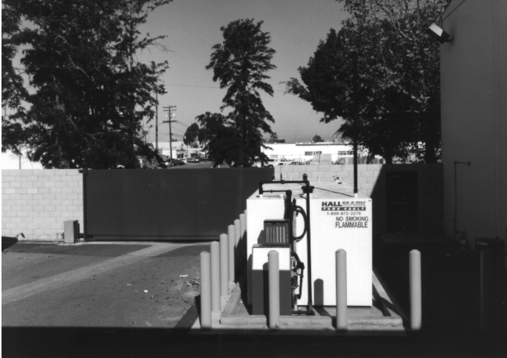
Figure 30. An above-ground tank was used to store M-85 at the demonstration site.
