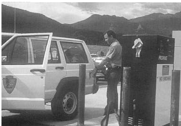
Rudy Marquez, heavy equipment mechanic and alternative fuel coordinator, Rocky Mountain National Park, with newly installed propane fueling station.
