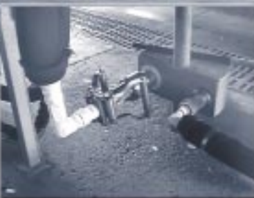
This docking station stores the LNG nozzles when not in use and serves as pre-cool circuit for the station. The liquid fill nozzle supplies 50 gpm.
