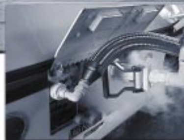
This docking station stores the LNG nozzles when not in use and serves as pre-cool circuit for the station. The liquid fill nozzle supplies 50 gpm.
