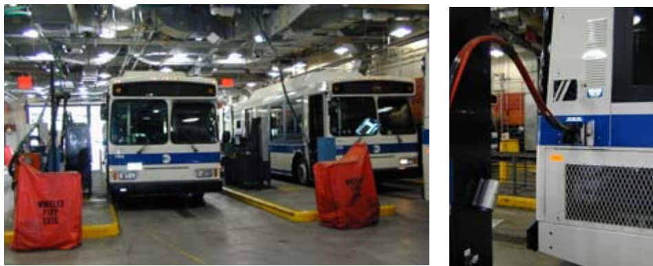
Figure 3. CNG Fuel Lanes at West Farms Depot
