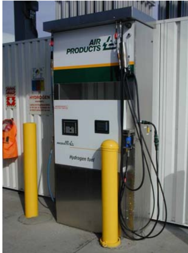
Figure 4. Hydrogen Dispenser
