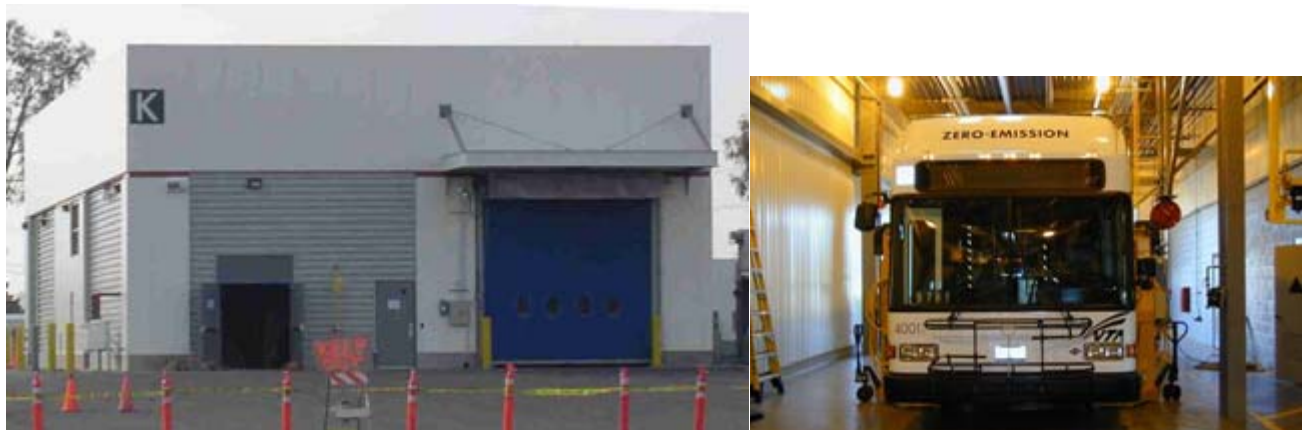
Figure 9. Maintenance Facility Used for the Fuel Cell Buses at VTA
