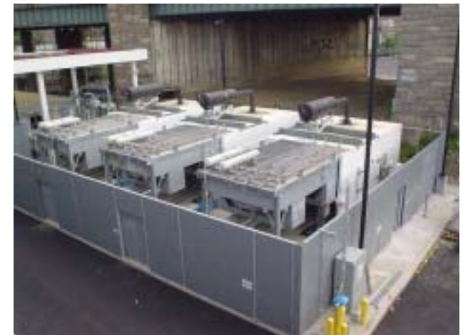
LACMTA Div 7, West Hollywood, CA. Close-up of compressor compound
