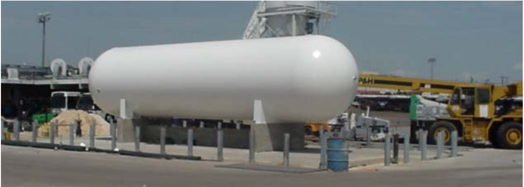
New 30,000 gallon propane tank being installed at San Antonio VIA Transit
