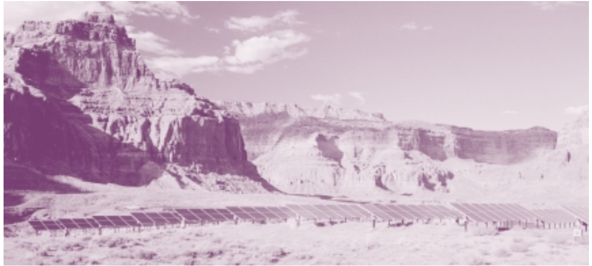
DANGLING ROPE MARINA, UTAH, UTILIZED A NEW GENERATION OF HYBRID PV POWER EQUIPMENT. THIS NEW TECHNOLOGY, COMBINED WITH THE DECLINING COSTS OF PV, CONTRIBUTES TO AN EXPANDING MARKET FOR LARGE-SCALE PV HYBRID POWER SYSTEMS.
