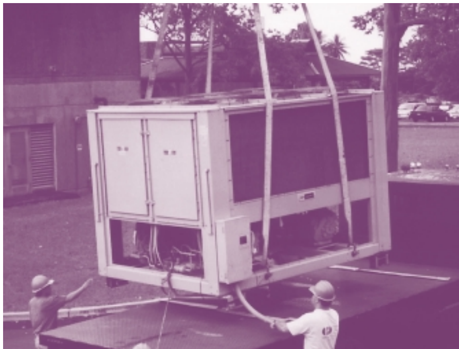
THE REBUILD HAWAII PROJECT PROVIDED FOR THE INSTALLATION OF A 400-TON VARIABLE SPEED CENTRIFUGAL CHILLER AT THE UNIVERSITY OF HAWAII.
