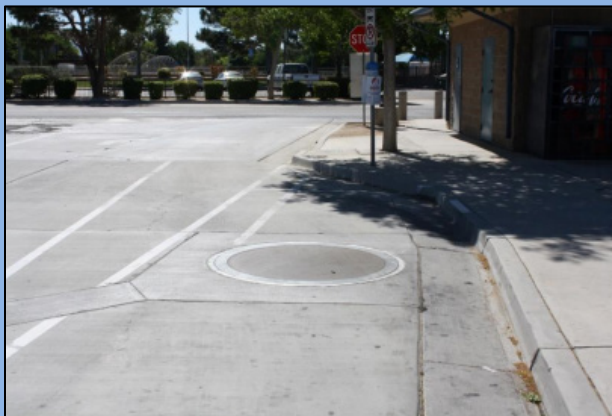
Figure 6. Wireless advanced vehicle electrification charging station for AVTA, embedded in the street
