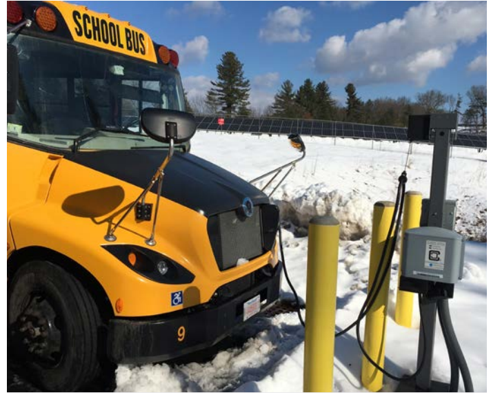
Battery-electric school bus in Massachusetts. Photo from Brian Foulds, Concord-Carlisle Regional School District, NREL 60242
