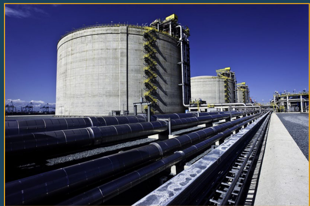
Figure 9. Storage tanks with heating pipes at the Port of Rotterdam (source: Port of Rotterdam n.d.[c]; photo by Eric Bakker ©).
