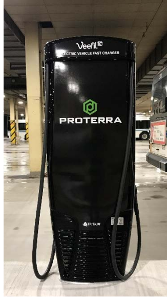
Figure 5. Electric vehicle supply equipment at DTA parking garage
