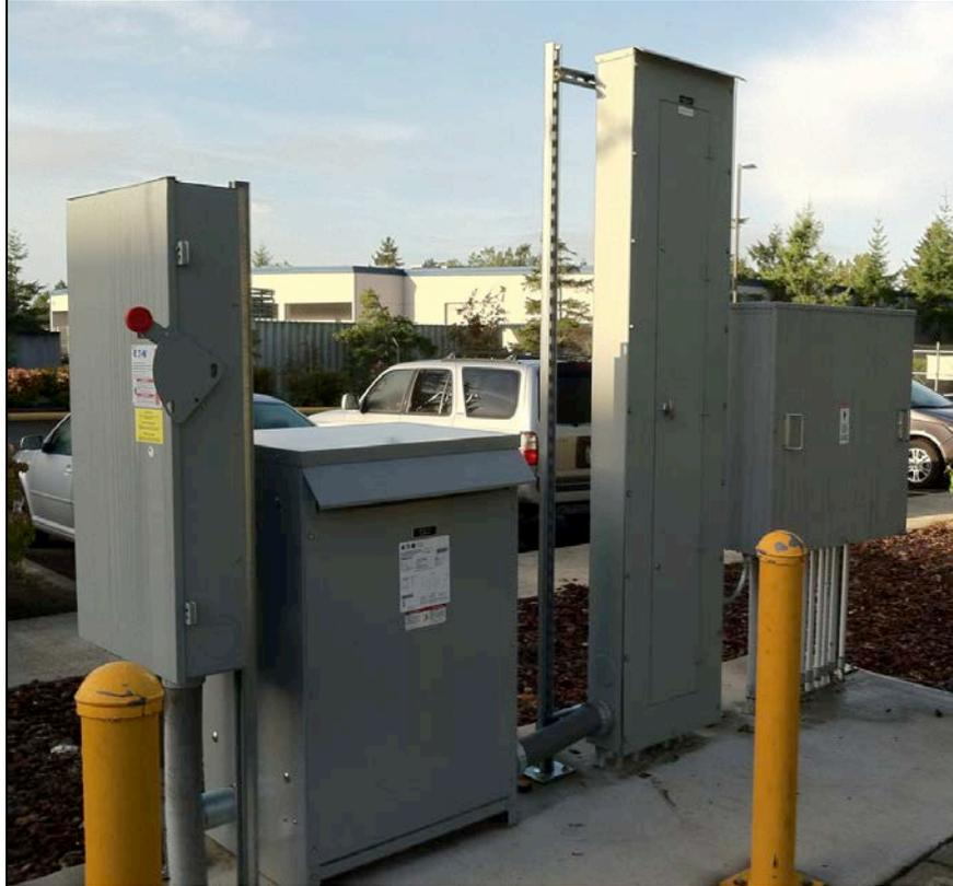
**Figure 24. EVSE power supply. From left to right: main disconnect, new transformer, load panel, and Chateau Energy Solutions monitoring equipment panel (Photo by Mike Simpson / NREL 29590)**
