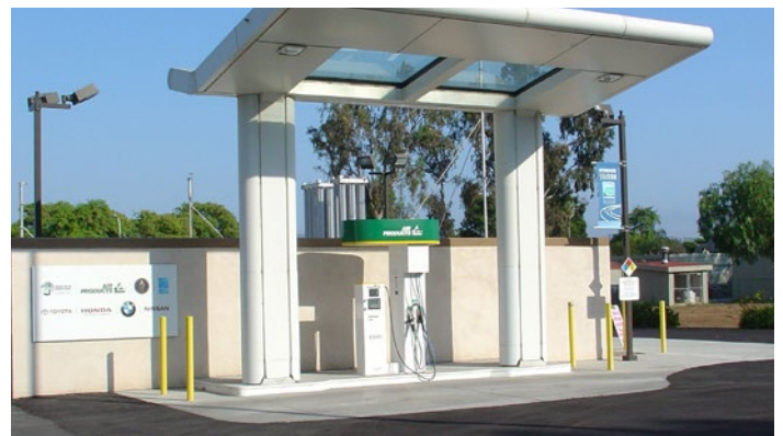
350/700 Bar Hydrogen Station and Dispenser. Photo by Keith Wipke, National Laboratory of the Rockies (NLR) 17316
