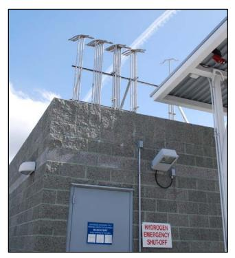
Figure 11. The vent stacks were raised above the level of the canopy
