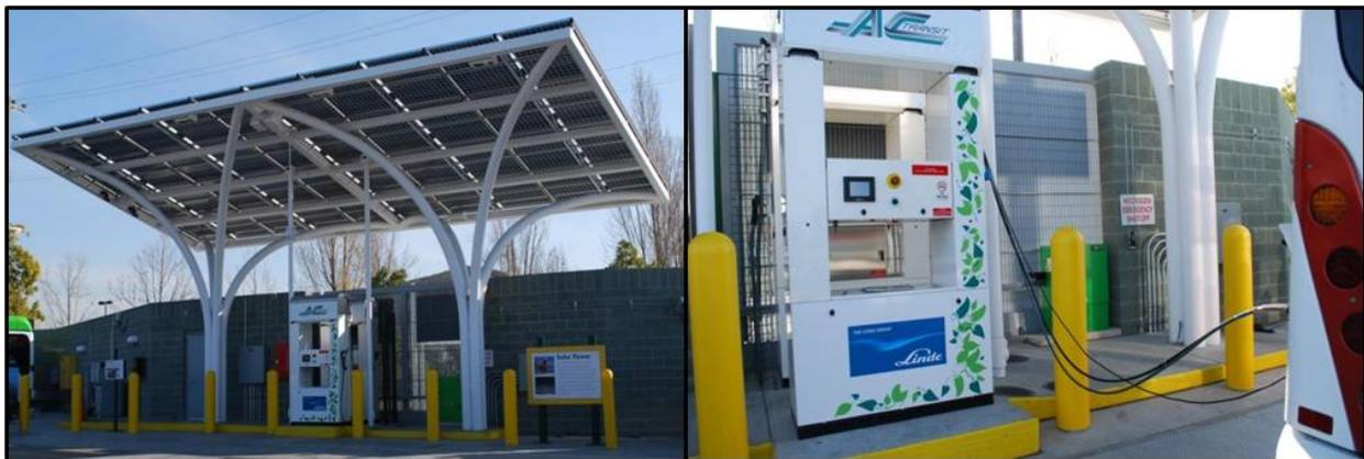
**Figure 8. Bus fueling at the Emeryville hydrogen station: fueling area (left) and close-up of the bus dispenser (right)**
