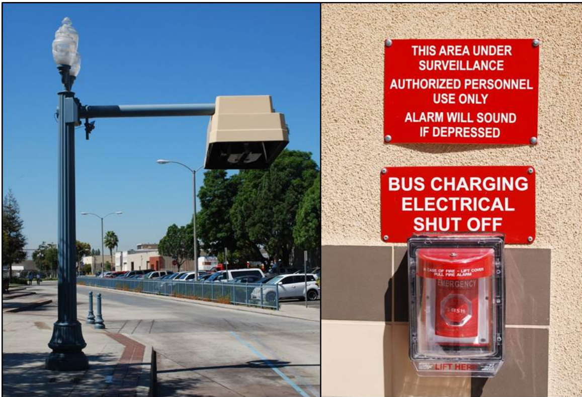
Figure 7. A charging head (left) and an emergency shut-off control (right) at the PTC
