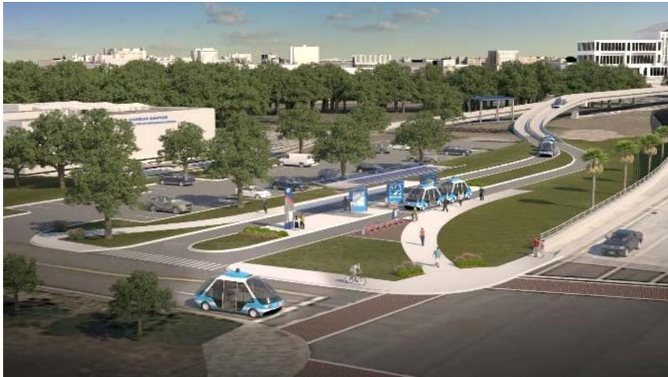
**Figure 3-14. Phase 2 transition to grade to allow U<sup>2</sup>C vehicles to operate along the BSIC AV lanes.**
