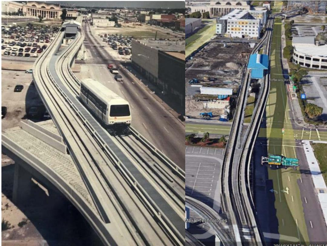
**Figure 3-12. Original Phase 1A segment showing 1989 automated people mover technology (left), and the retrofitted small monorail beam currently in place today (right).**
