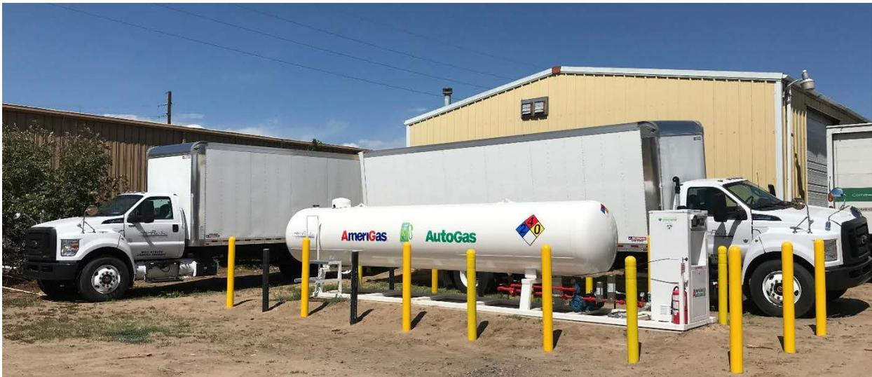
**Figure 2. Photo of the propane fuel station installed at the Hi Pro truck depot**
